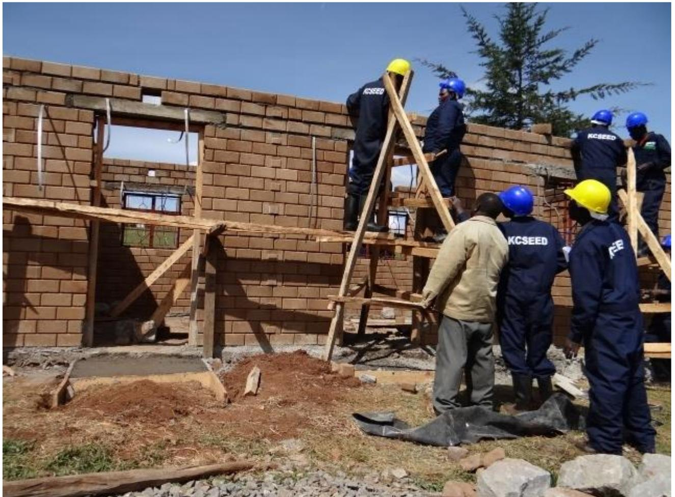
Figure 1 the first building to be put up using hydra form technology
